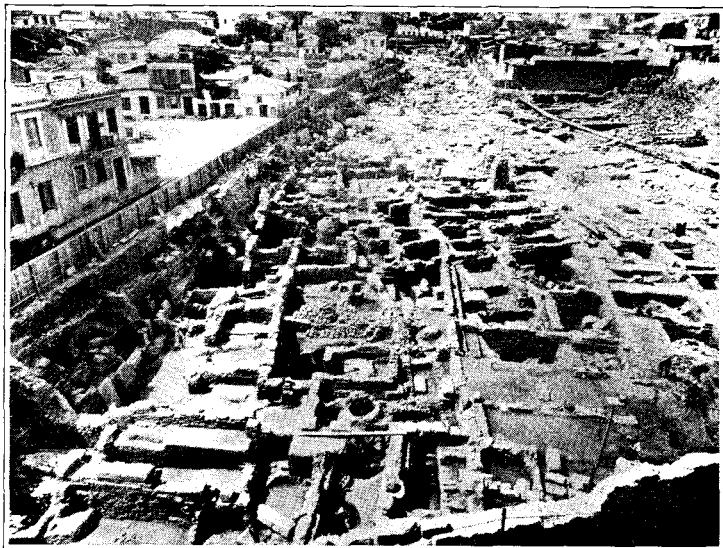
FIG. 178. Excavations being carried on in the ATHENIAN MARKET PLACE (Agora) by the AMERICAN SCHOOL AT ATHENS
